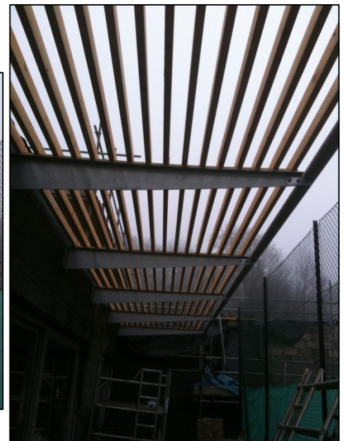
Supporting Steelwork View from Below
