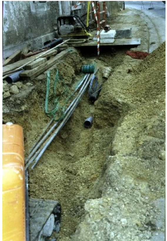
Vacuum Sewer being installed alongside other services
