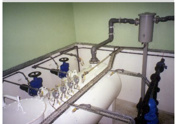
Vacuum Vessel and associated equipment
