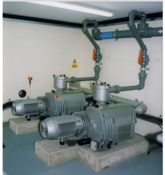
630m 3 /hr Vacuum Pumps Installed
