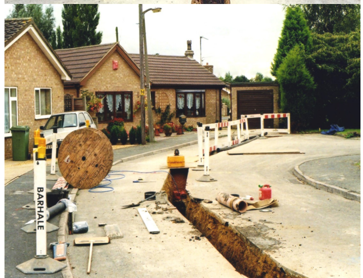
Preparing the trench for the vacuum main to be laid
