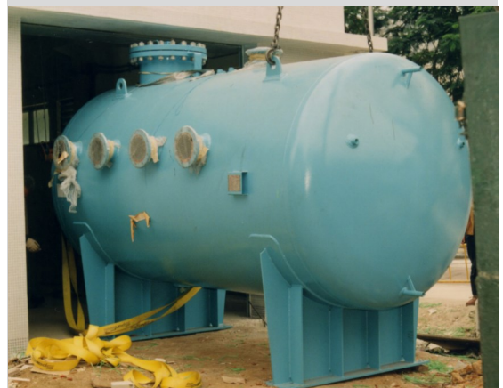
Vacuum Vessel being installed
