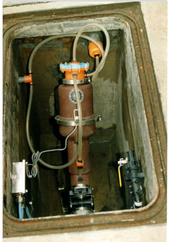
Interface Valve in bespoke chamber
