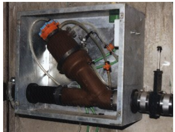
Interface valve mounted in wall cabinet.
